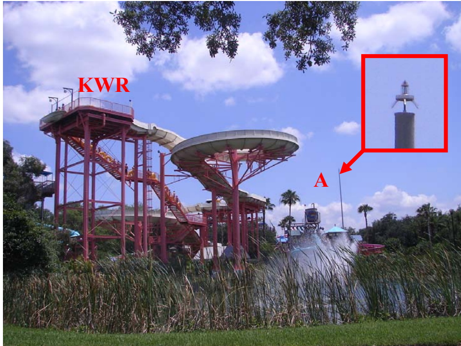
Fig. 5: Position of lightning rod A in relation to the KWR water slide.
