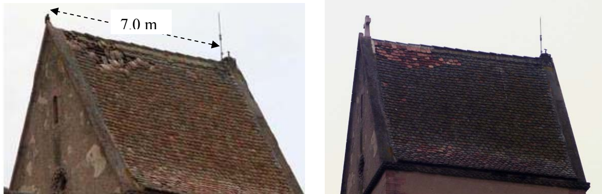
Fig. 16: The bell tower with the (missing) damaged stone cross (left) and the new stone cross installed a year later (right). The ESE lightning rod is installed on the opposite side of the roof.
